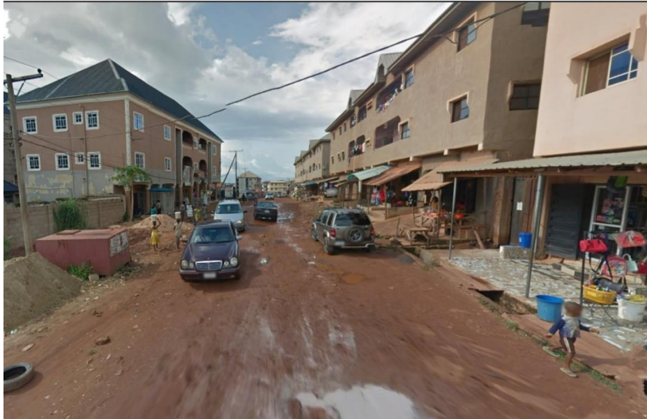
Plate 2. Violated setback in front of the yard at Ologo Road, Achara Layout Enugu. Source: Authors fieldwork (June 23, 2023)
