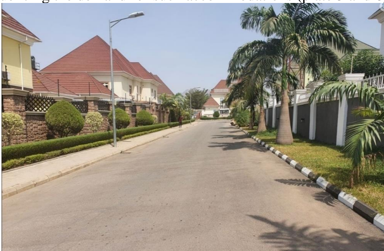
Plate 5. Residential layout with landscaping elements at Fidelity Estate, G.RA Enugu. Source: Authors fieldwork (June 23, 2023)
