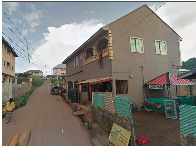
Plate 3. Building structure encroaching to the road at Ekowa Street, Achara Layout Enugu. Source: Authors fieldwork (June 23, 2023).
